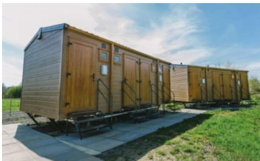
The toilet and shower block near the camping field.
